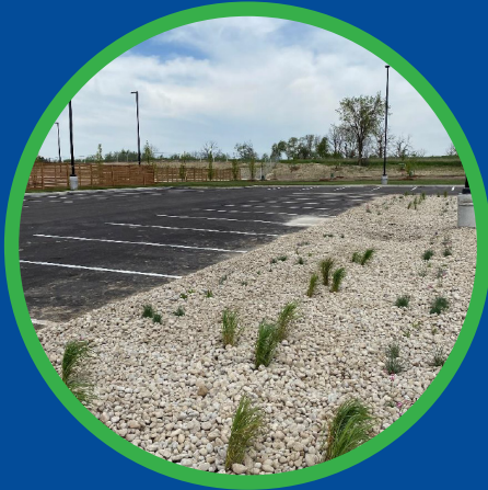
PARKING WITH LOW IMPACT DEVELOPMENT BIOSWALE
