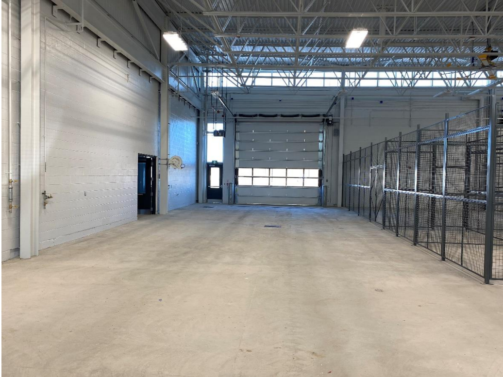
CPRC service bay and storage cages
