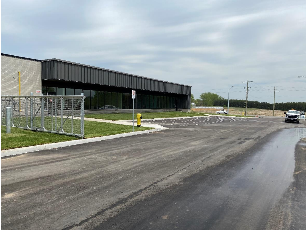
South elevation service drive viewing toward Woodbine Avenue
