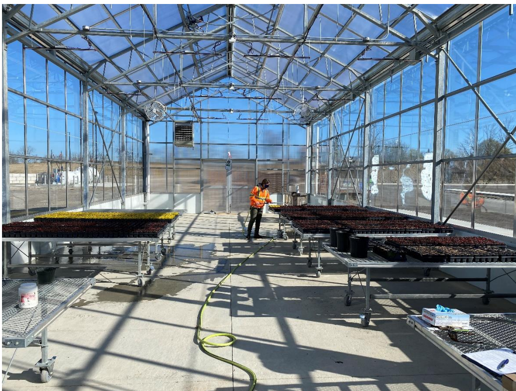
Environmental controlled greenhouse with planter tables
