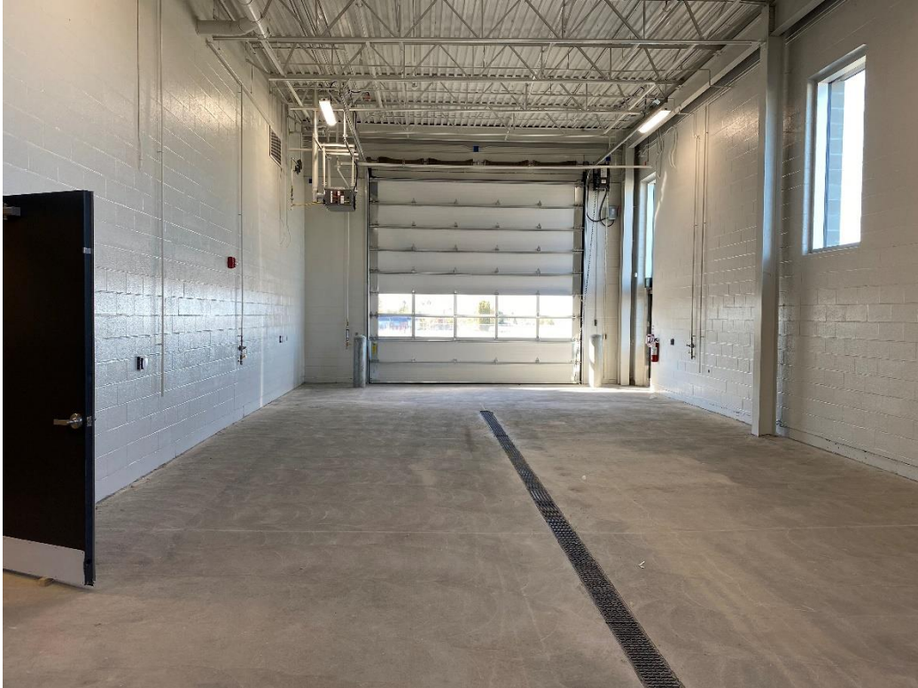
Wash service bay
