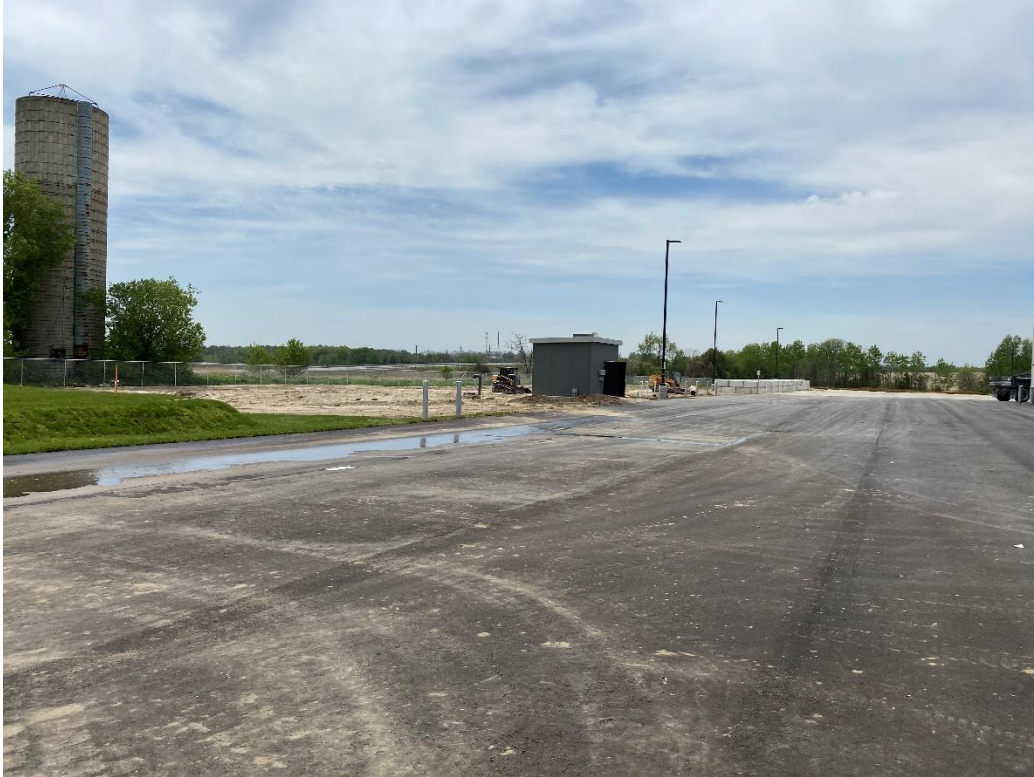
South elevation fire safety system pumphouse and material storage bays
