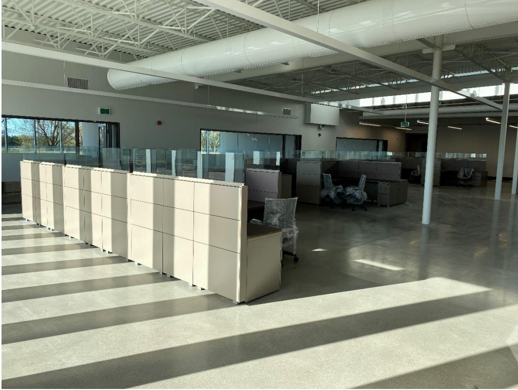
Administrative area open office work stations
