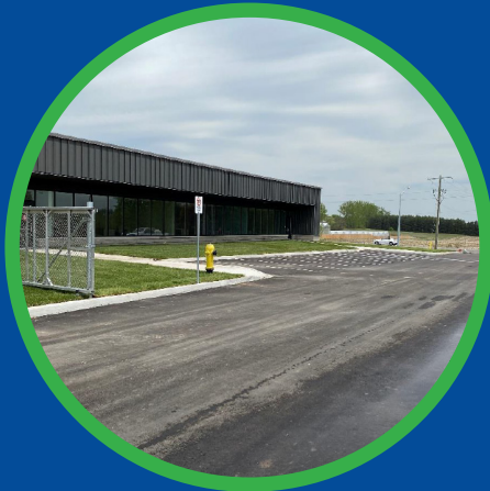
SERVICE DRIVE ENTRANCE AT WOODBINE AVE.
