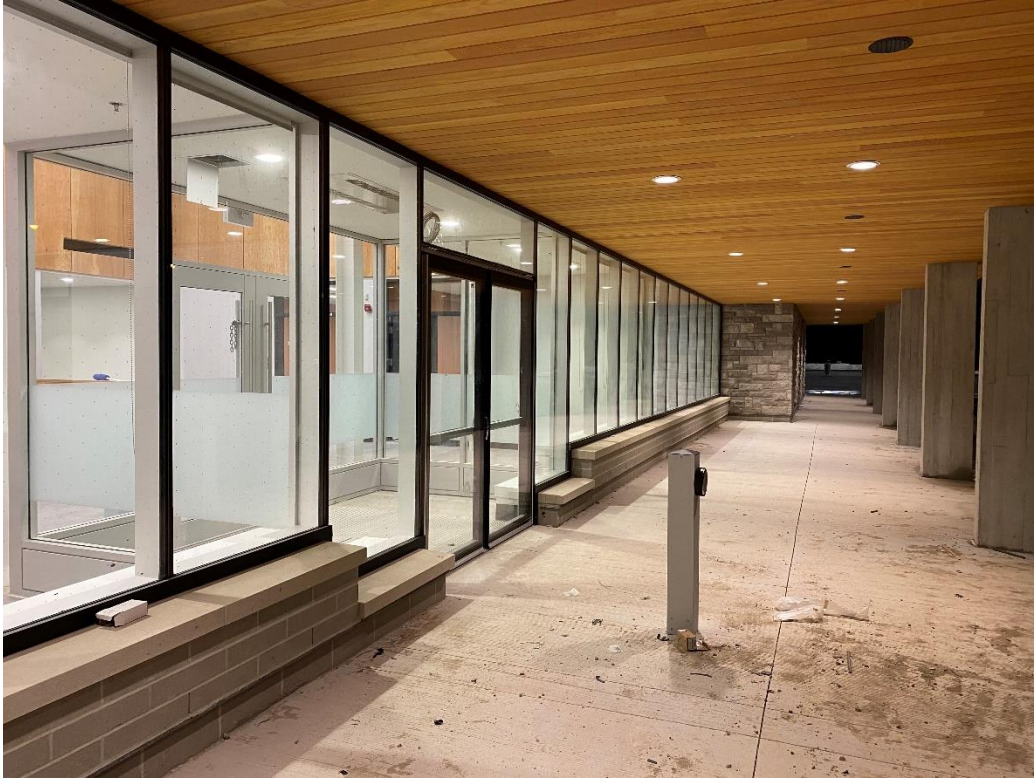
East elevation public entrance connected to public parking
