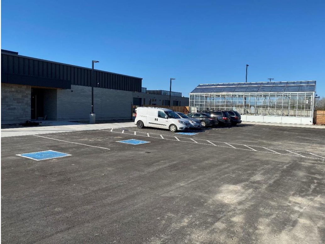
North elevation parking and employee field operator entrance
