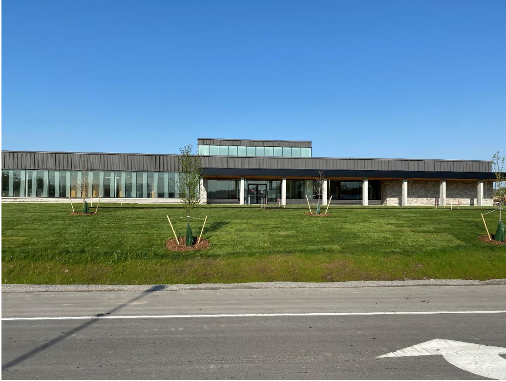
Front of house east elevation view from Woodbine Avenue
