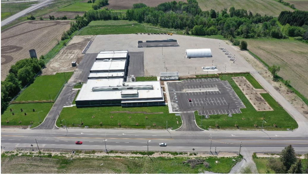
Aerial view east elevation from Woodbine Avenue
