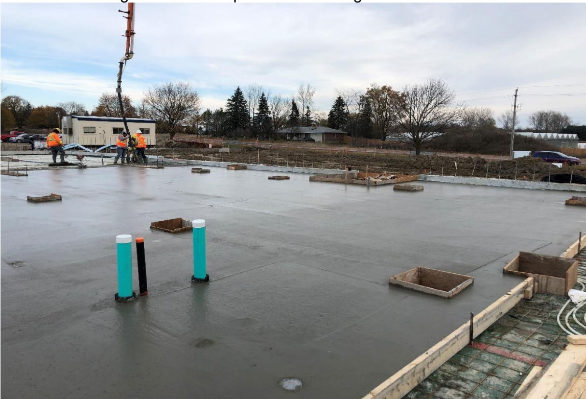
Slab on grade concrete pour EOC and administration meeting rooms
