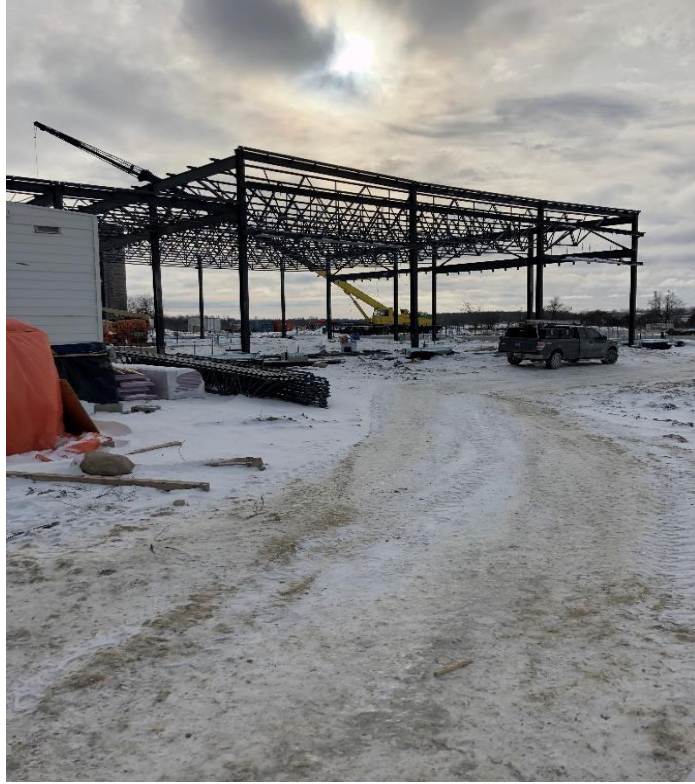
Structural steel Water & CPRC service bays
