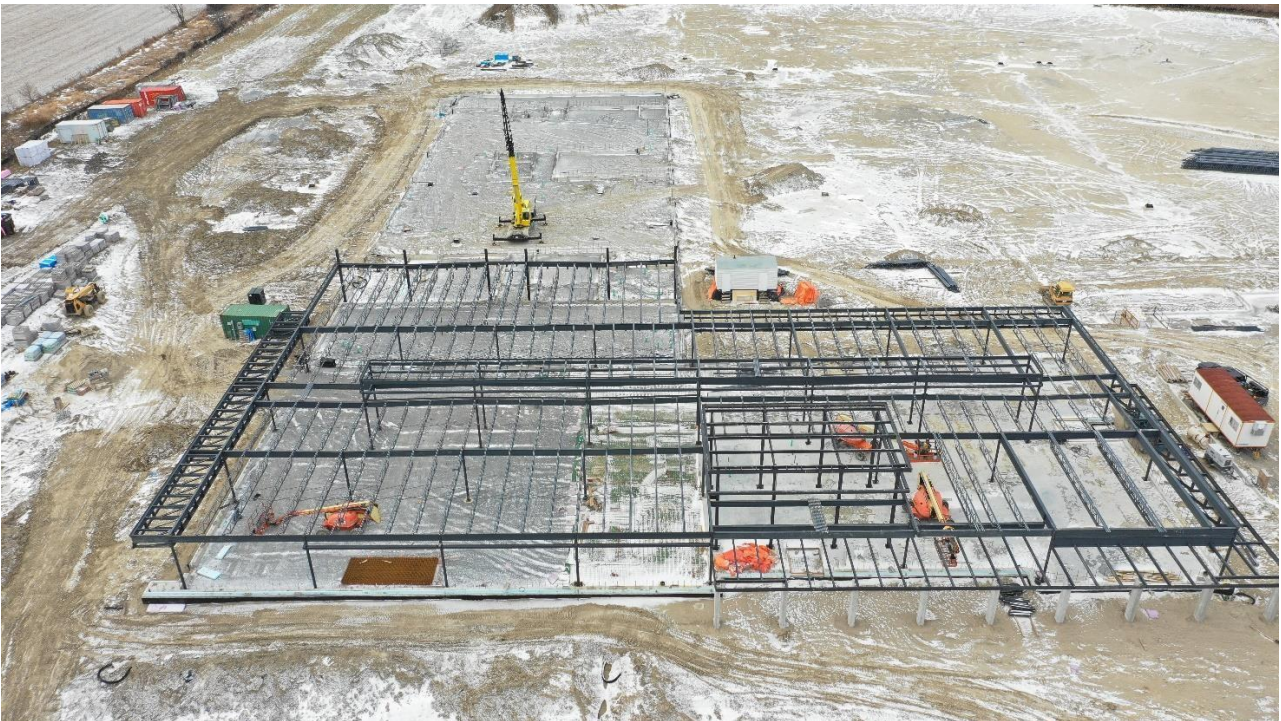
Aerial view looking west of foundation & structural steel footprint December 2019
