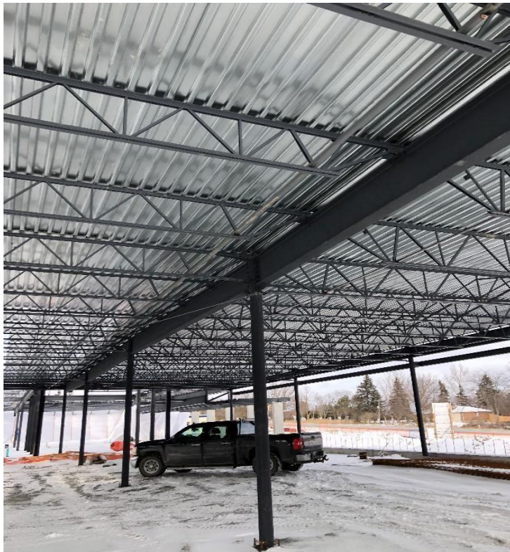
Steel decking placed, installed along administration area
