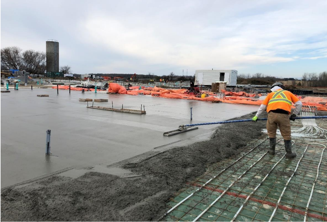
Slab on grade concrete pour and finishing north administration area
