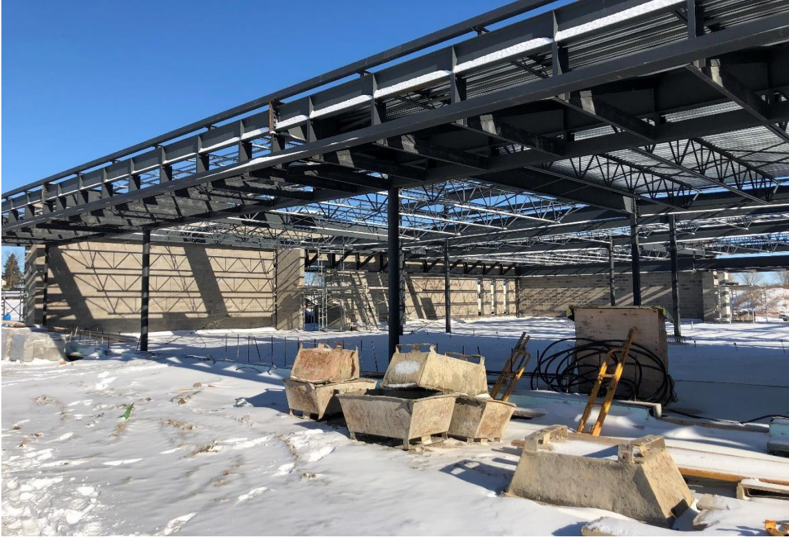
Steel columns, beams, trusses and decking along north administration area
