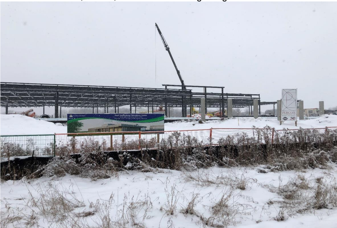
Facility east elevation view of structural steel
