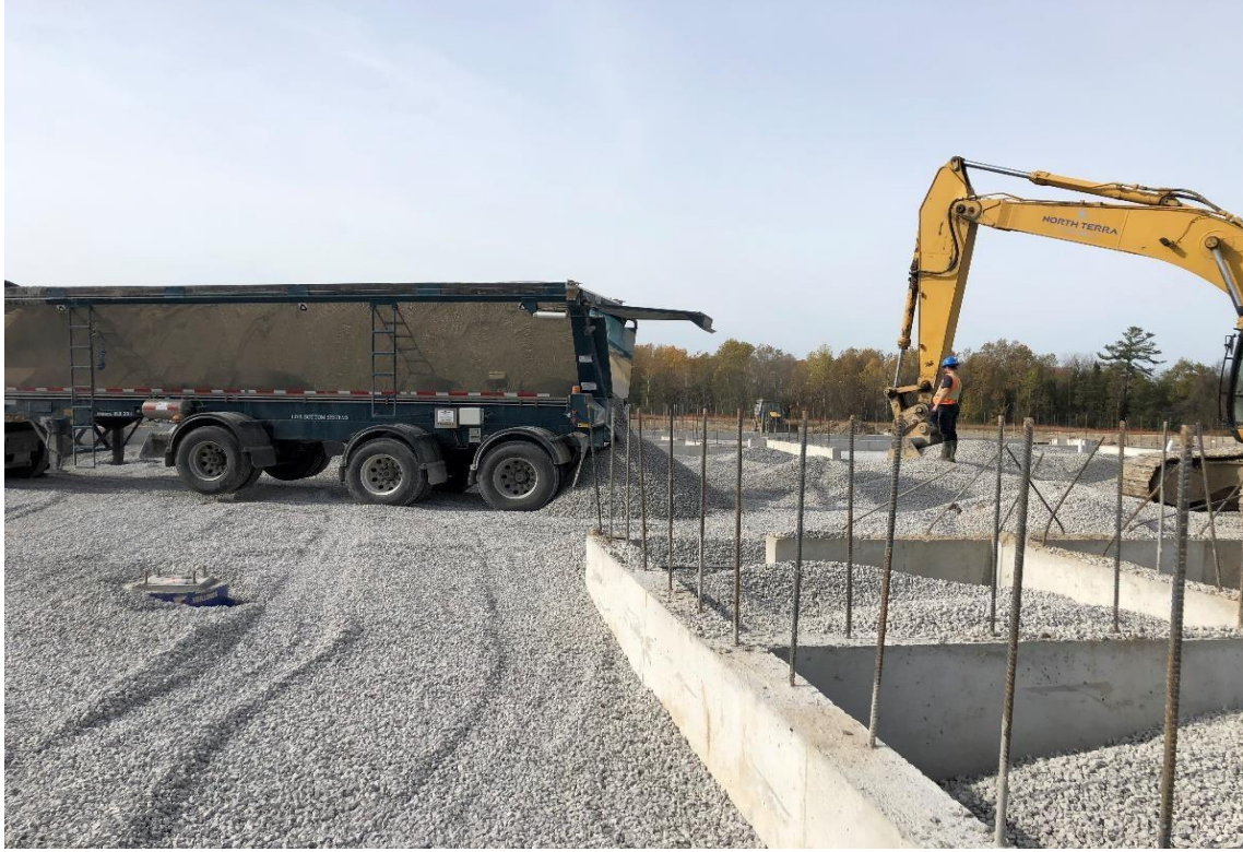
Placement of foundation stone service bays
