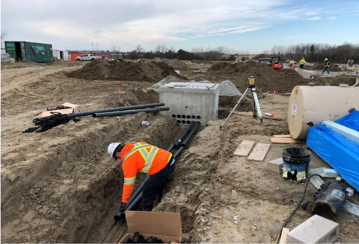
Installation of primary electrical duct bank to service facility
