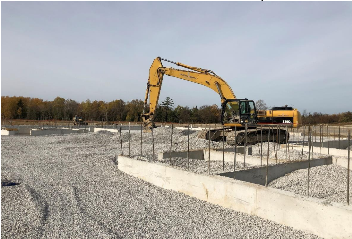
Foundation stone placement along interior foundation walls of service bays
