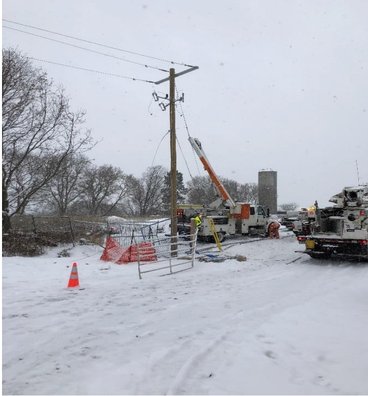
Hydro One installation to service facility
