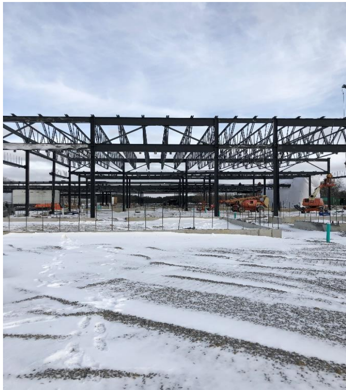
Viewing east of Water & CPRC service bays
