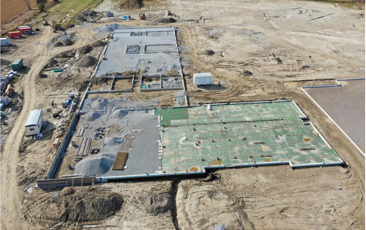
Aerial view looking west of foundation footprint October 2019
