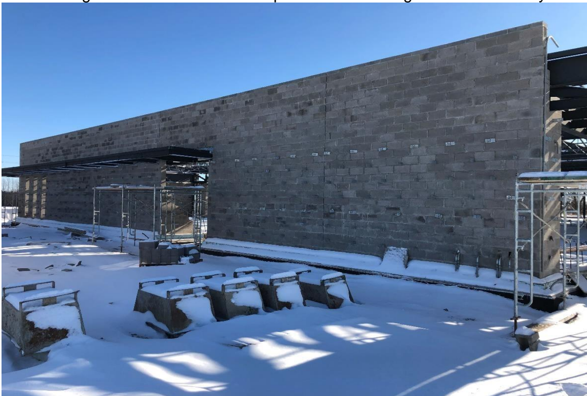
Masonry wall north elevation for EOC and lunch room
