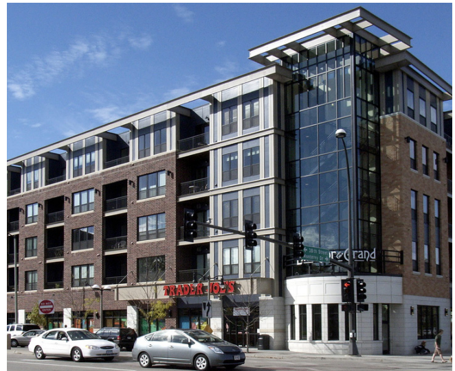
Articulation of the facade with various materials and offsets.
