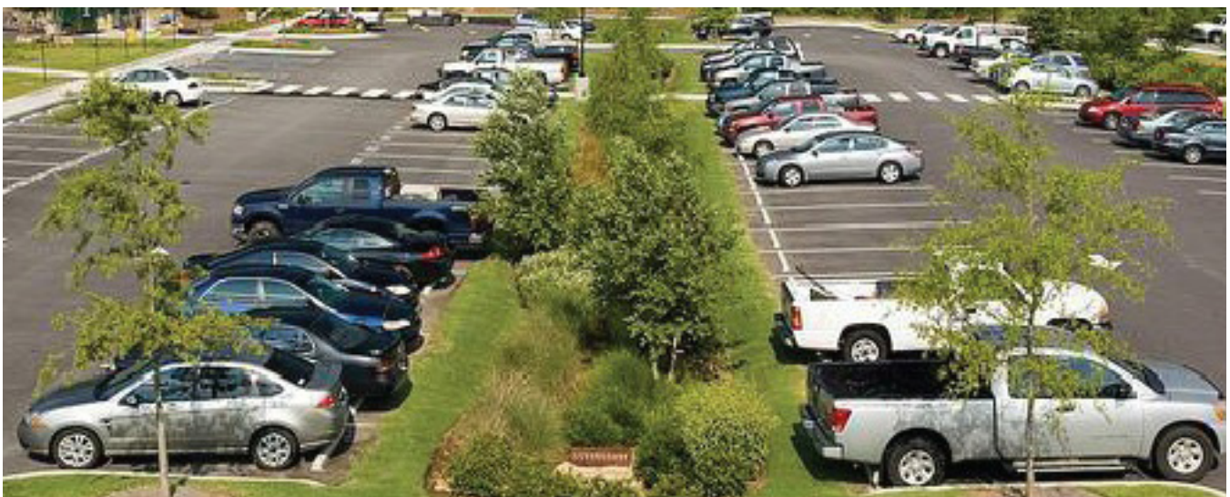
Example of a parking lot that incorporates planting strips for as a stormwater management strategy.
