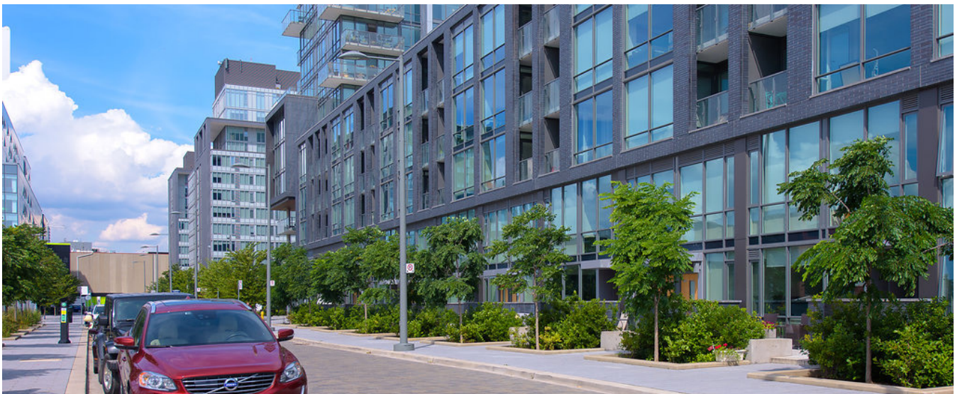
Example of a building with inset balconies to minimize shadowing the balconies below.
