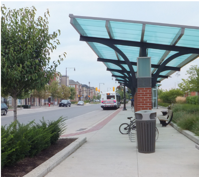
Canopy to provide shade, seating, waste receptacles, and bicycle parking at a transit stop.
