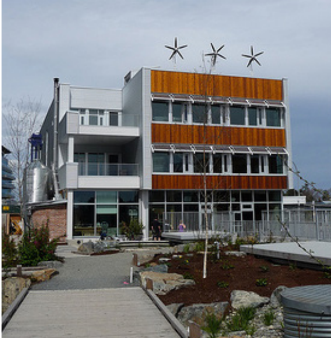
Wind turbines on the roof of an office building.
