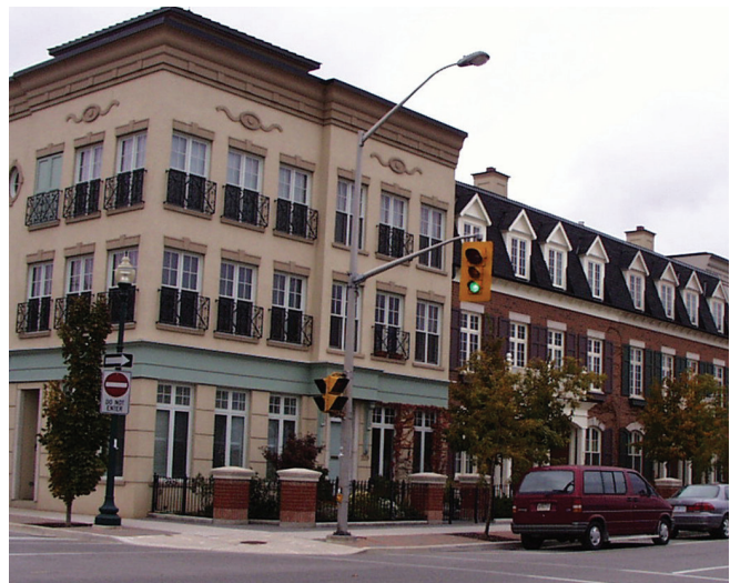
A consistent building setback frames the street..
