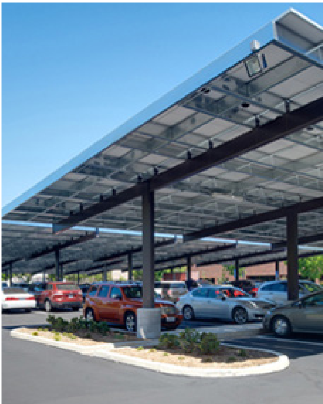
Solar canopies in surface parking lots.
