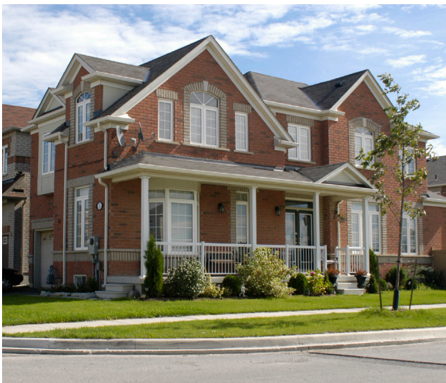
Single detached dwelling with upgraded side elevation.
