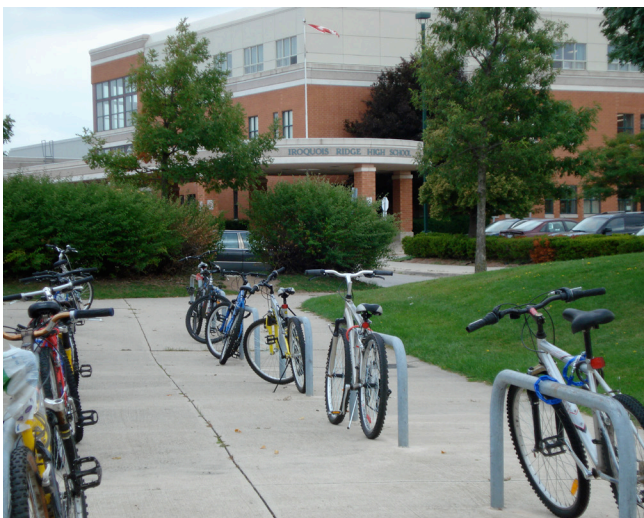
Bicycle parking is provided in close proximity to the front entrance of the school.
