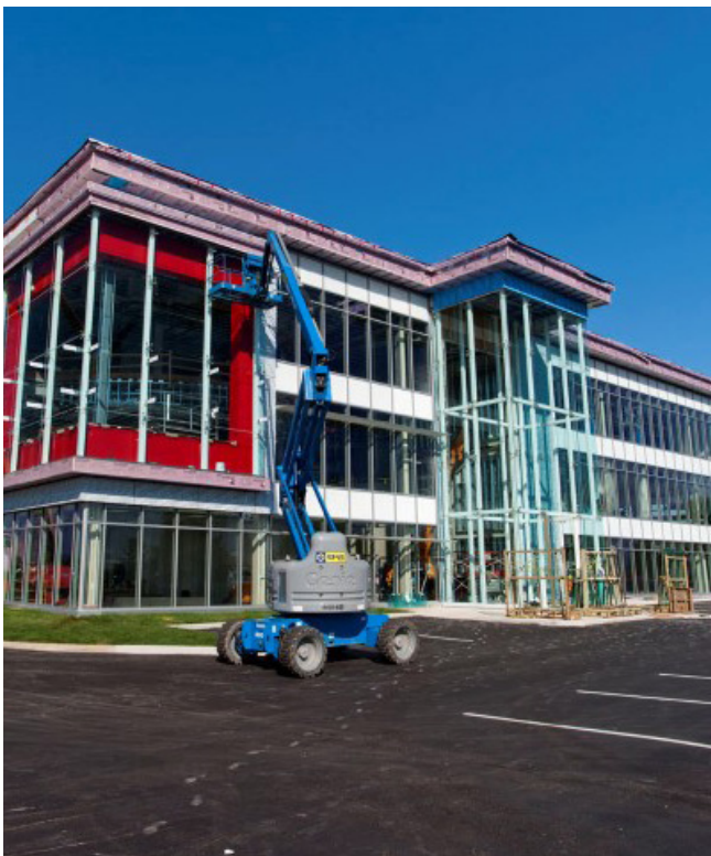
Construction of an employment building.
