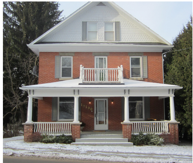
Existing residential dwelling that illustrates entry elements such as porches and generous overhangs to articulate front elevations at entrances.
