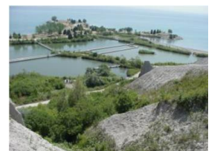
'End of Pipe' Controls
