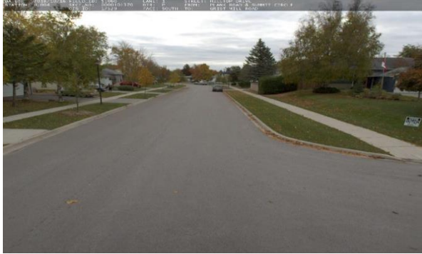
Figure 37: Images of Pavement Condition Very Good
