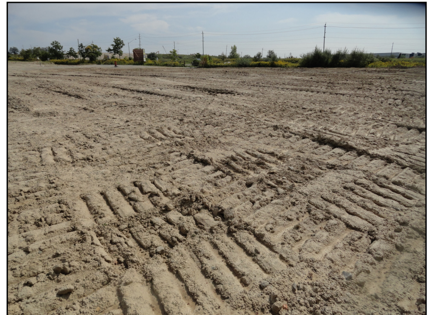
Photograph 8. Southeast view of Site (CVC_1), devoid of natural vegetation cover, topsoil stripped, filled and graded in 2021 and 2022 by permit
