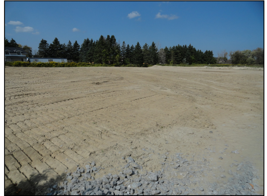
Photograph 6. Northwest view of Site (CVC_1) from construction road access entrance off of Green Lane East, devoid of natural vegetation cover, topsoil stripped, filled and graded in 2021 and 2022 by permit
