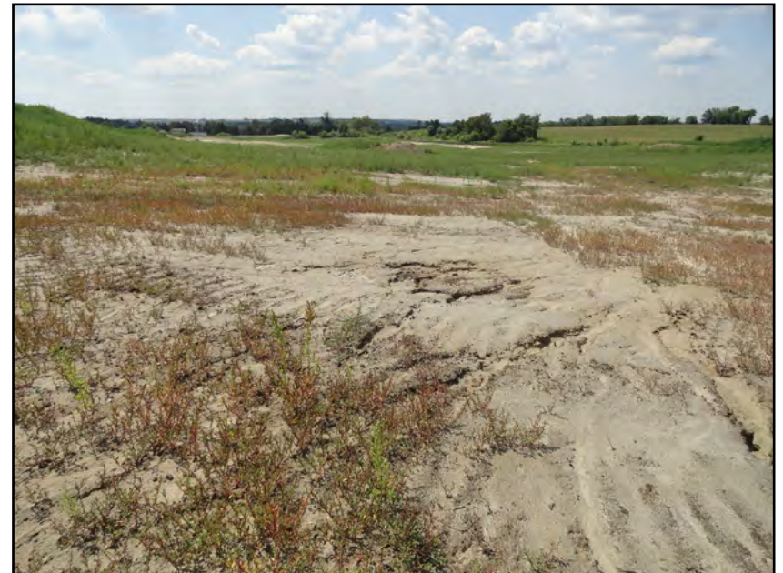
Photograph 12. Westward view of tableland agricultural cropland (OAGM1), showing topsoil removal (0.3m) and topsoil stockpiles as permitted under the Earthworks Agreement
