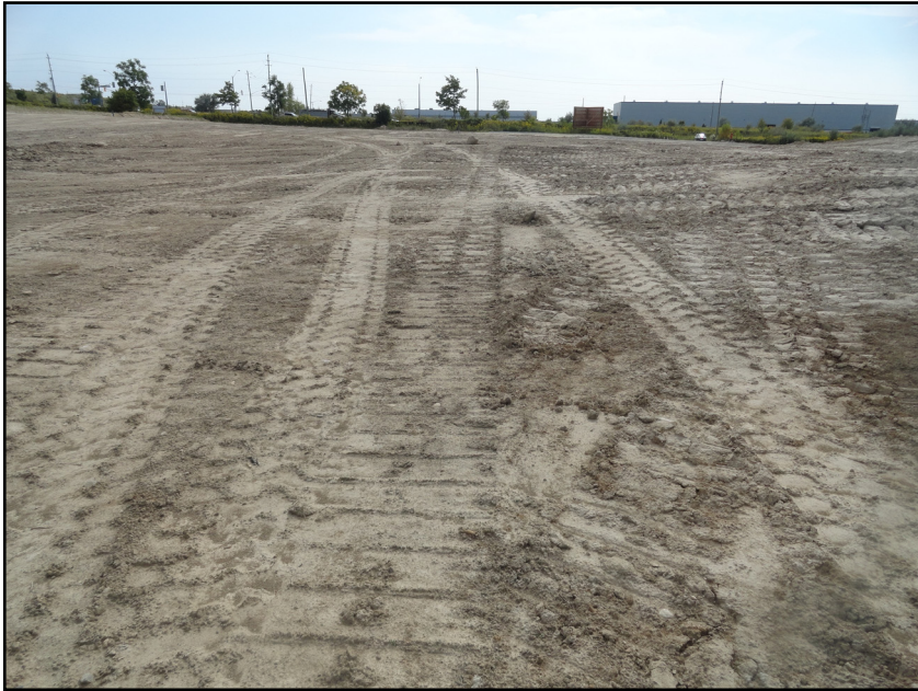
Photograph 9. Southward view of Site (CVC_1), devoid of natural vegetation cover, topsoil stripped, filled and graded in 2021 and 2022 by permit
