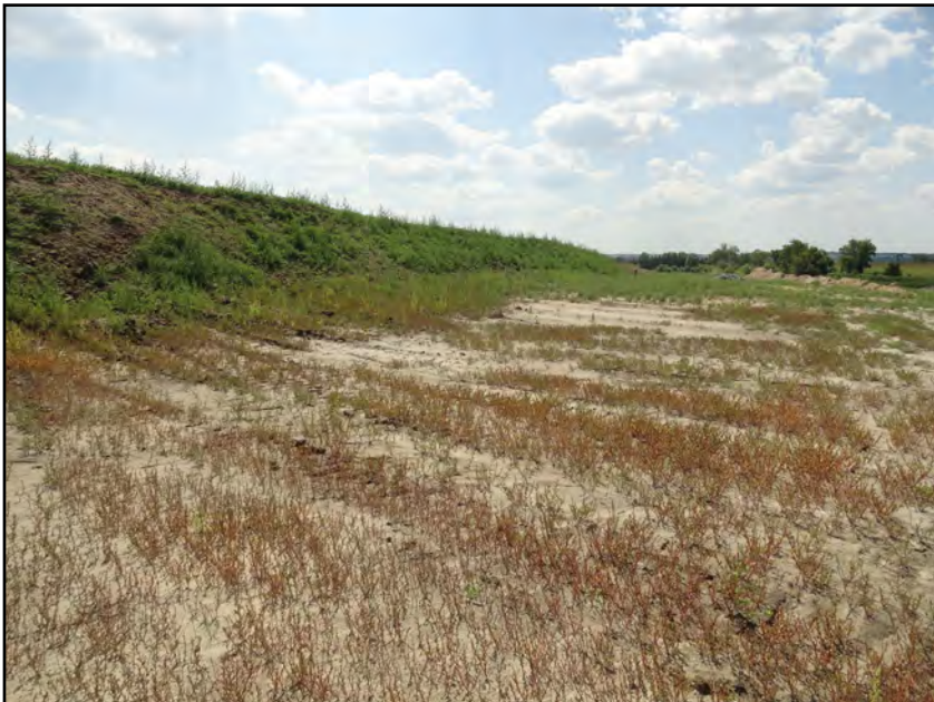
Photograph 11. Northwest view from east end of property, showing tableland agricultural cropland (OAGM1) removal and stocking piling of 0.3m of topsoil, as permitted by Earthworks Agreement
