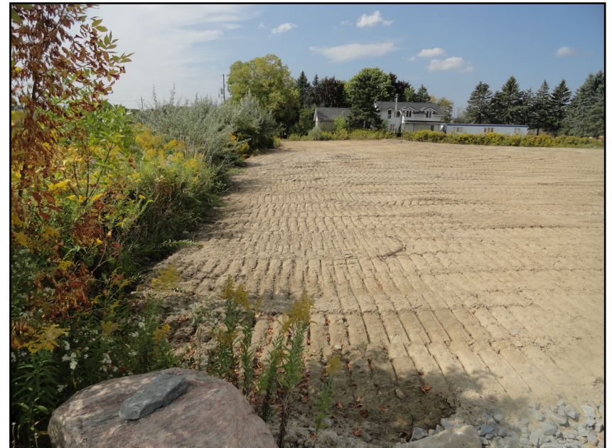
Photograph 4. Westward view from construction road access of previous residential lot in southwest corner of Site (CVC_1), cultural and natural vegetation removed, topsoil stripped, filled and graded in 2021 and 2022
